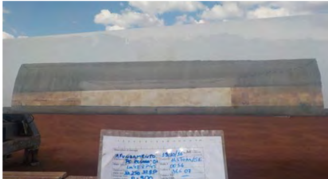
Small to Large Sandwich Repairs
