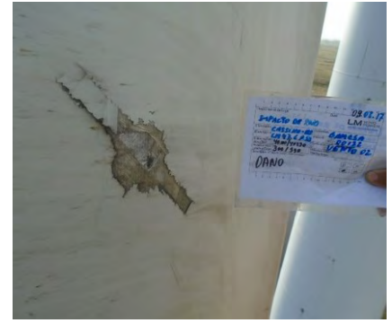
External and Internal Lightning Repairs
