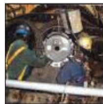
Flow Sleeve Removal
