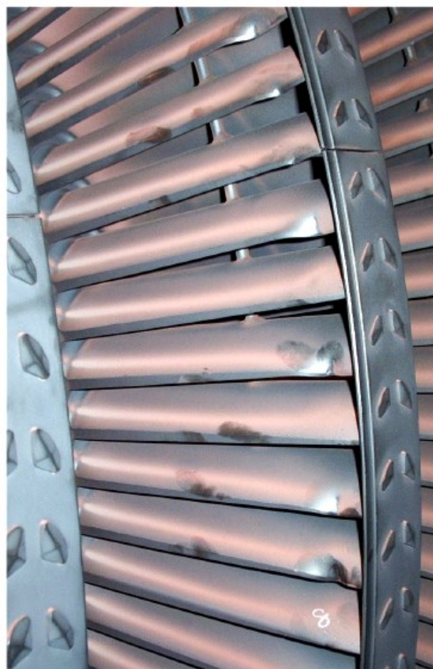
Fig 1: Blade damage on an IP rotor
