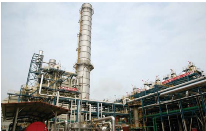
Figure 9. 9E plant located in China using syngas.
