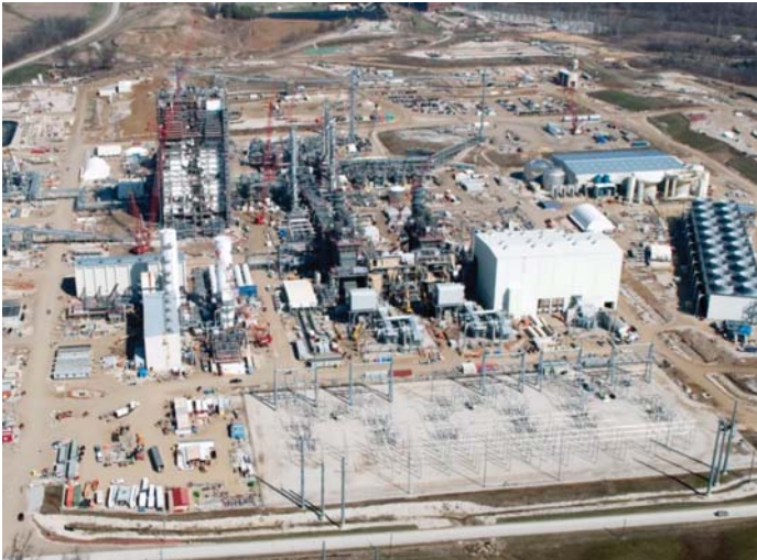
Figure 11. Duke Edwardsport IGCC plant (2011).
