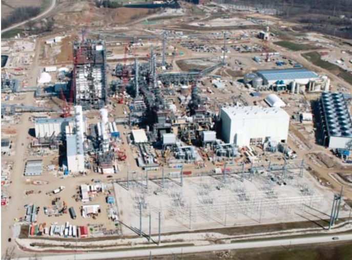
Figure 11. Duke Edwardsport IGCC plant (2011).
