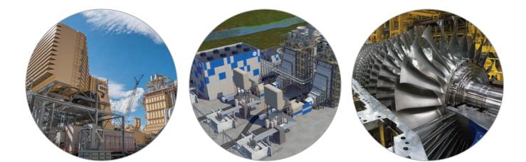
GE's 7HA.03 gas turbine is the highest capacity 60 Hz gas turbine with a rating of over 430 MW and combined cycle outputs of 640 MW (1x1) and 1,282 (2x1).
