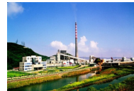
Zhoushan Power Plant MV Switchgear+Transformers, $2MM
