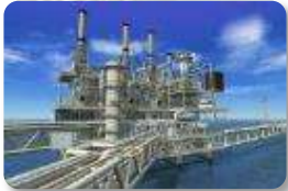
Upstream onshore & offshore gas
